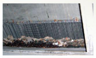
Bar rack with a fine spacing; the bars have a streamlined tear drop profile resulting in low head loss and avoiding jamming; Jagtap's screens are unimpaired by grit and gravel
